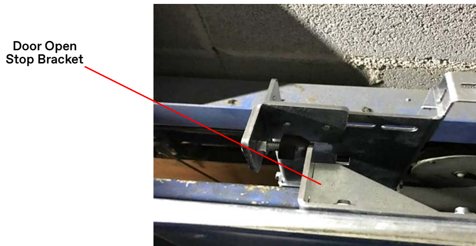
Figure 7 - Door Open Stop Bracket Installation
