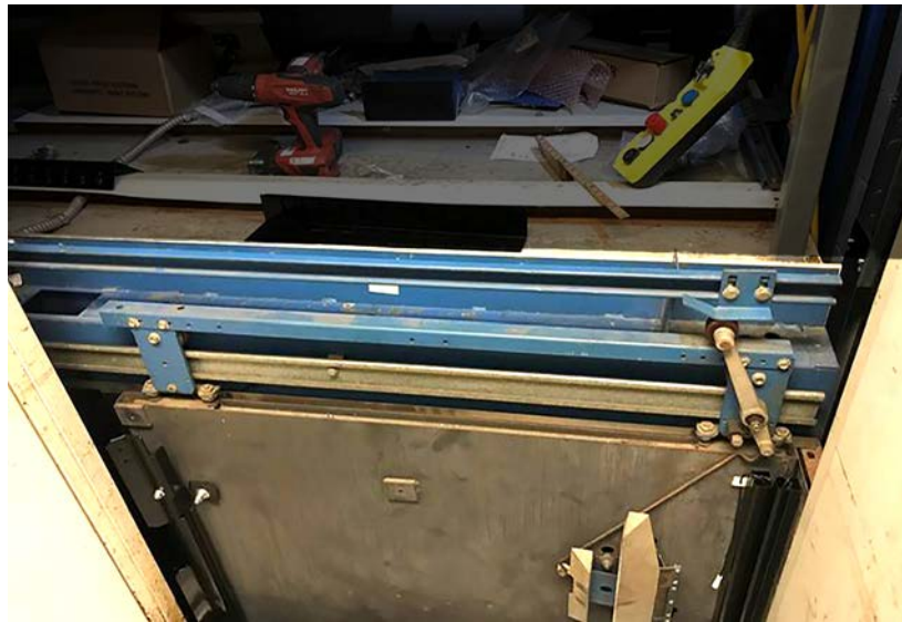
Figure 1 - Existing Door Operator Drive Components Removed
