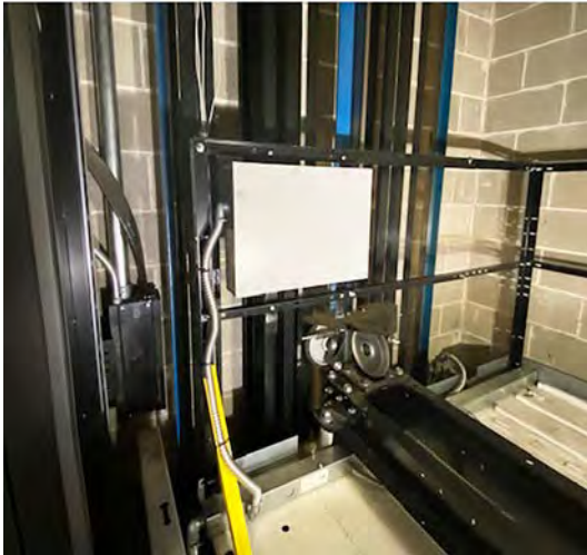
Car Top Box Mounted on Car Top Rail
